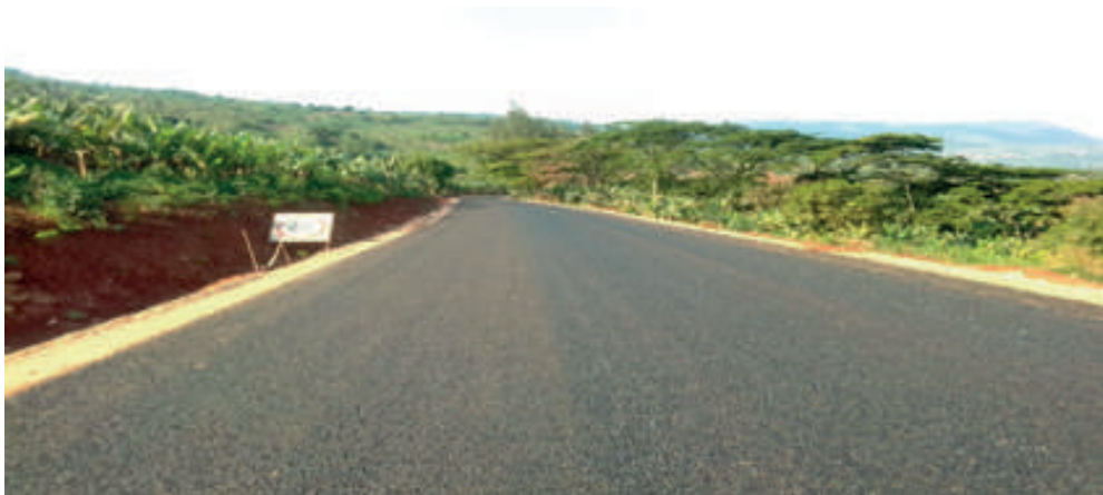
Completed restoration works on the Kopa-Jopa Road in Chimanimani
