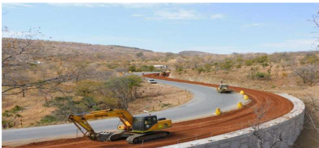
Upgrading works on the Harare–Chirundu Road
