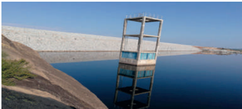
Newly constructed Causeway Dam
