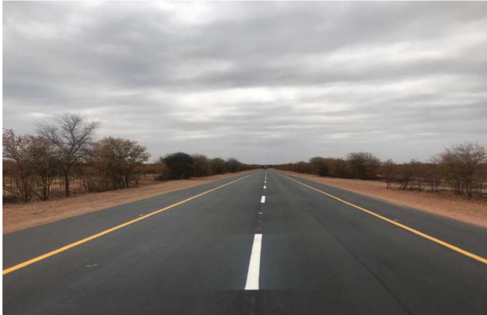
Completed section of the Harare-Masvingo-Beitbridge Road
