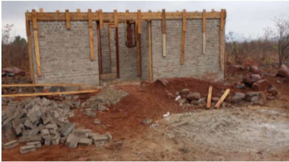
Houses being constructed for families affected by Cyclone Idai at West End Farm, Nedziwa
