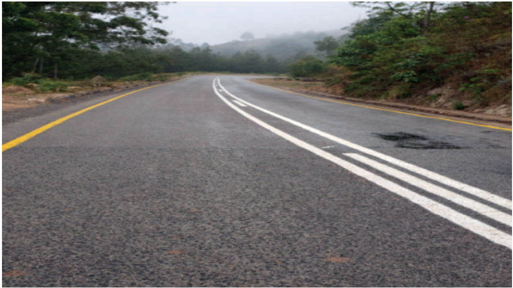
Completed restoration works on the Skyline-Chimanimani Road
