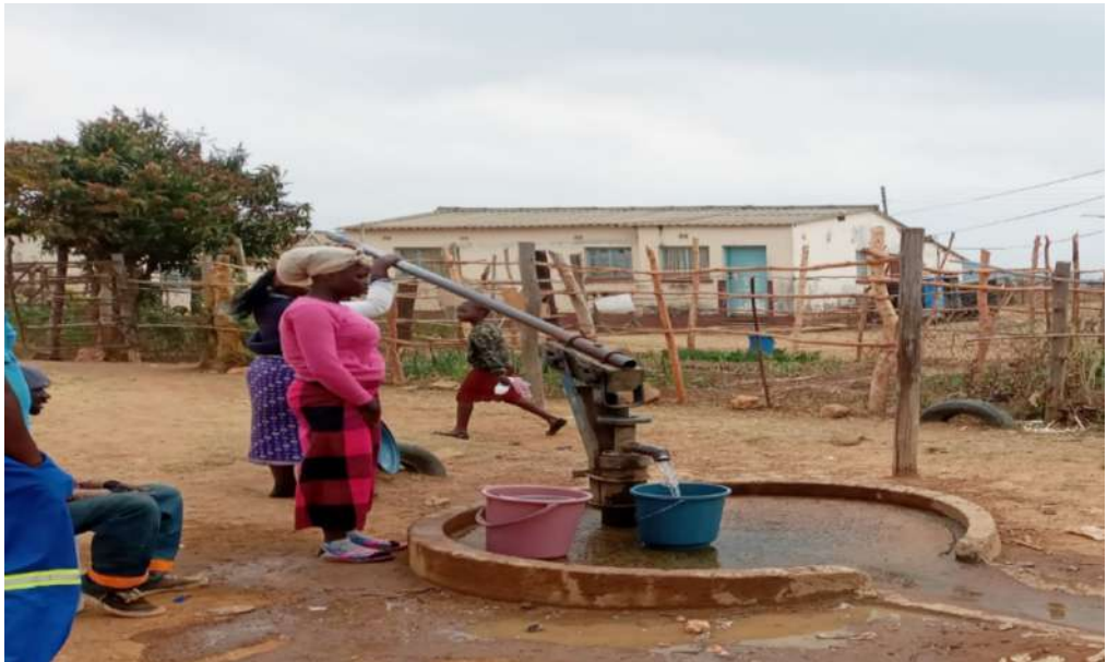
Rehabilitated borehole at Howard High School, Mazowe District
