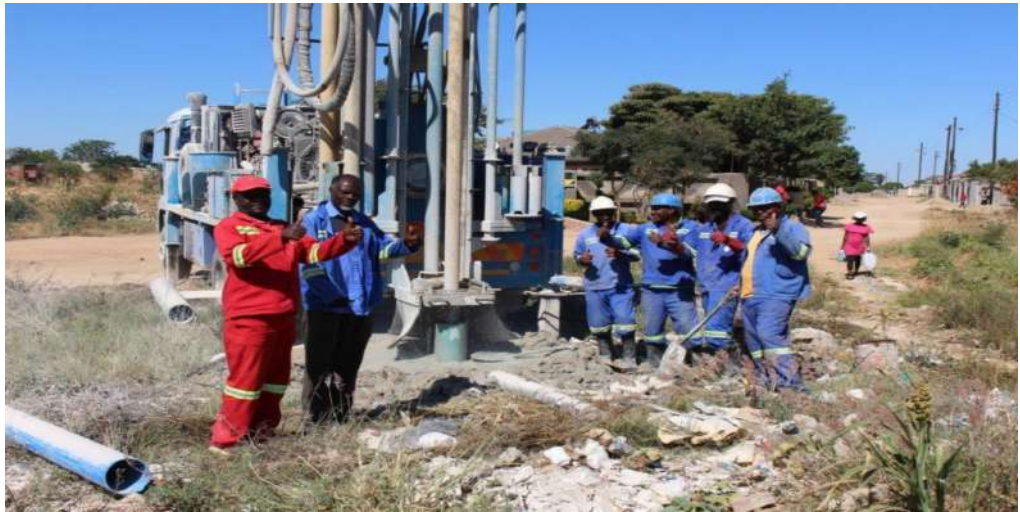
ZINWA personnel drilling a borehole in Chitungwiza
