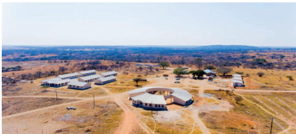
Completed structures at Makumimavi Primary School
