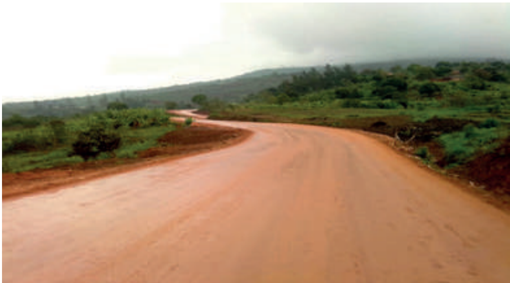
Restoration works in progress on the Kopa-Jopa Road in Chimanimani
