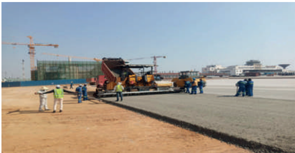
R. G. Mugabe International Airport: Construction of the new A380 apron next to domestic terminal
