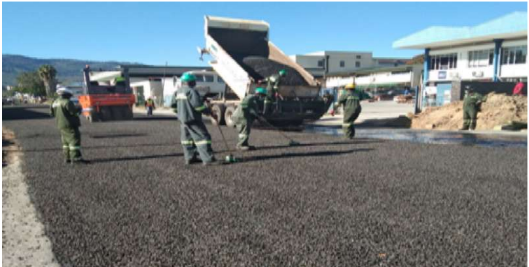
Roadworks being undertaken in Mutare's CBD, funded by the Road Fund
