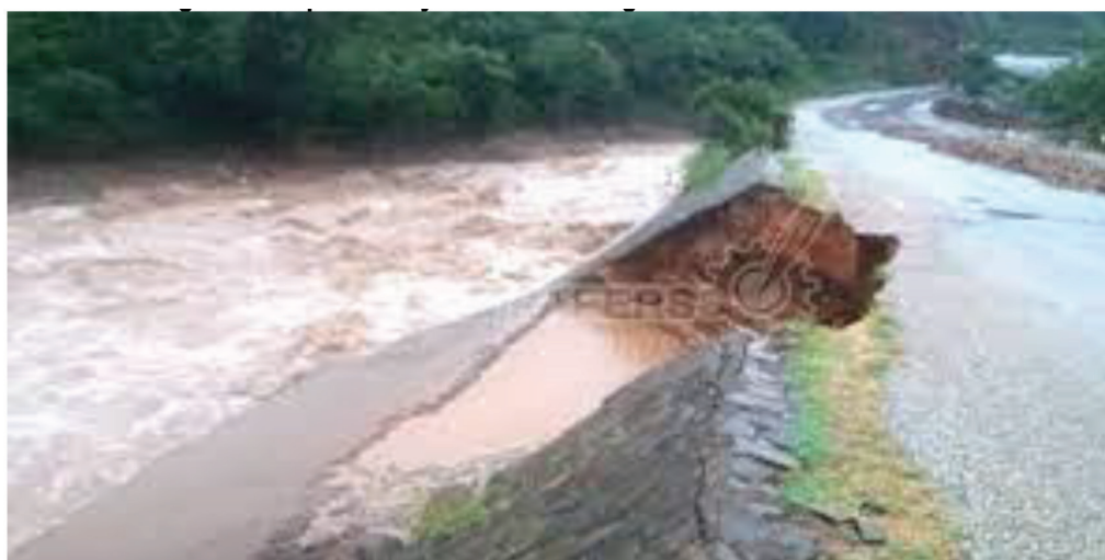
Figure 6: Impact of Cyclone Idai along Mutare Chimanimani Road
