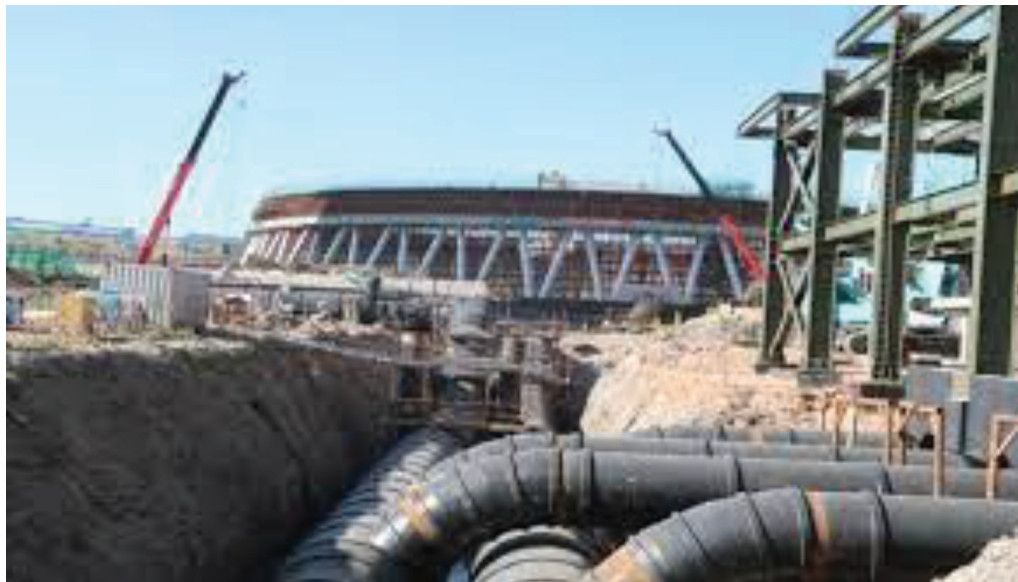
Figure 10: Hwange 7 & 8 Expansion Project
