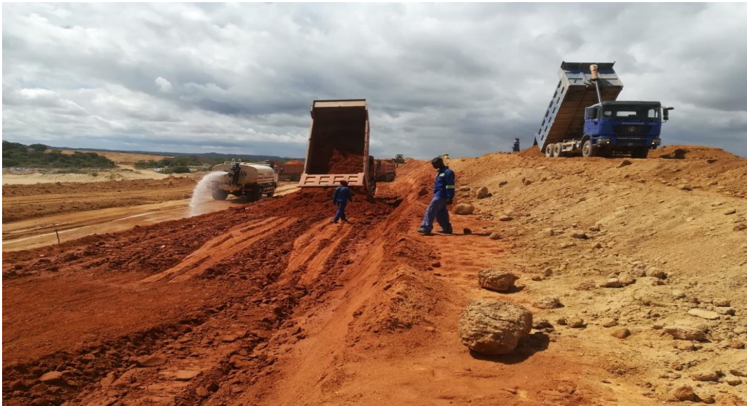
Causeway Dam - main dam placing of fill and core material in progress
