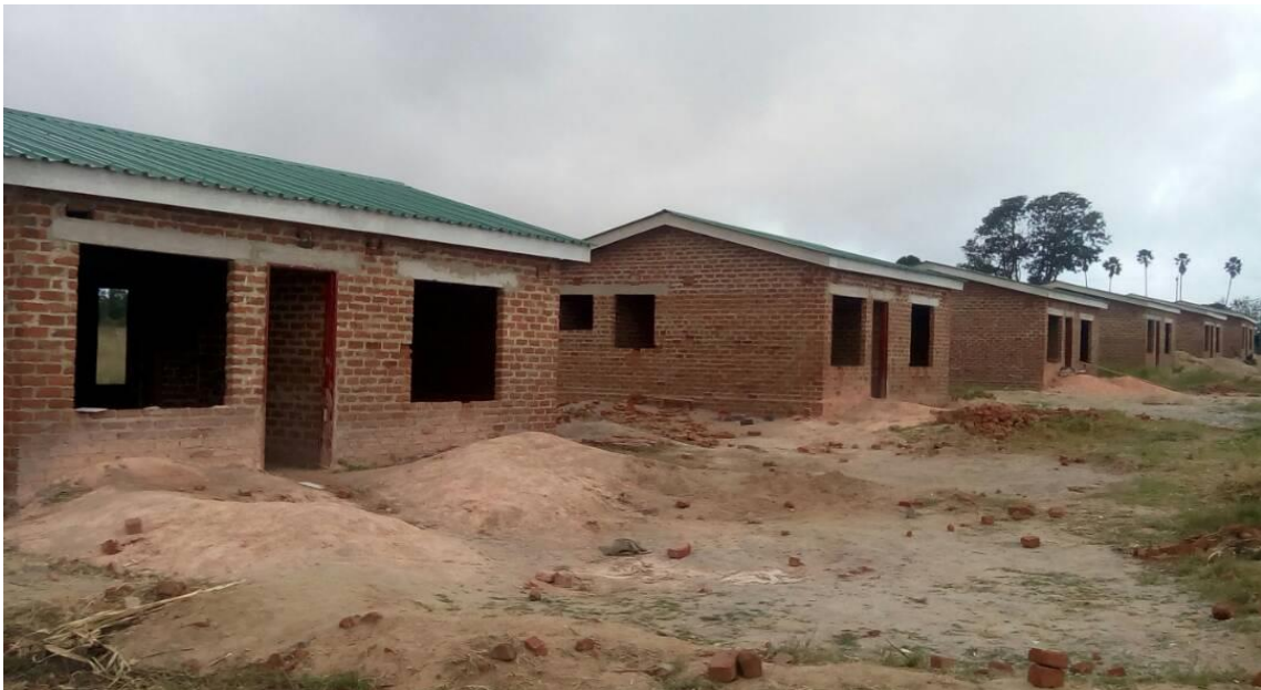
ZPCS staff houses under construction
