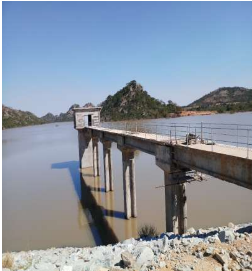
Upstream View of Marovanyati Dam
