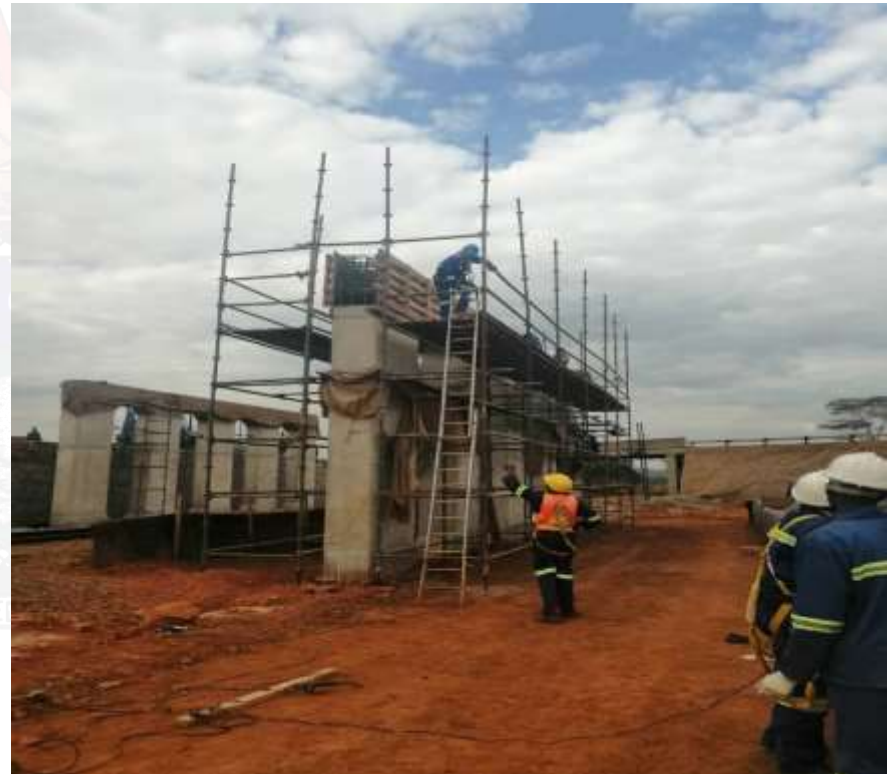
Ongoing works on the Norton Road Over Rail Bridge
