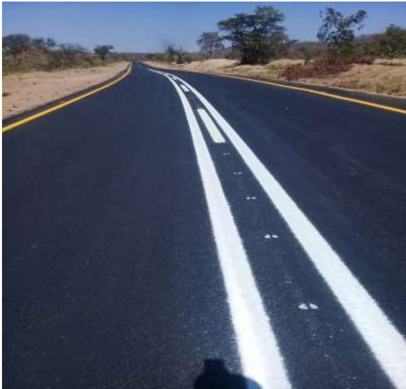
Completed section of the Bindura-Matepatepa Road
