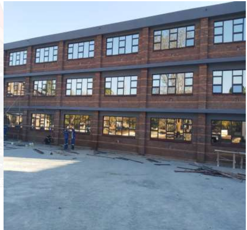
Final touches to the Innovation Hub at the University of Zimbabwe
