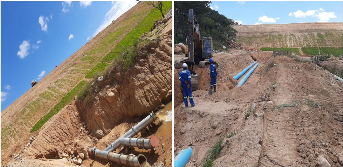
Figure 31: Connection and laying of pipes from the dam to the water treatment plant as well as irrigation outlets at Chivhu
