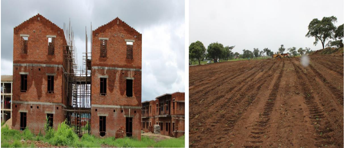
Figure 35: Construction of Dzivarasekwa Flats and site clearing for construction of flats at Senga Messenger's Camp
