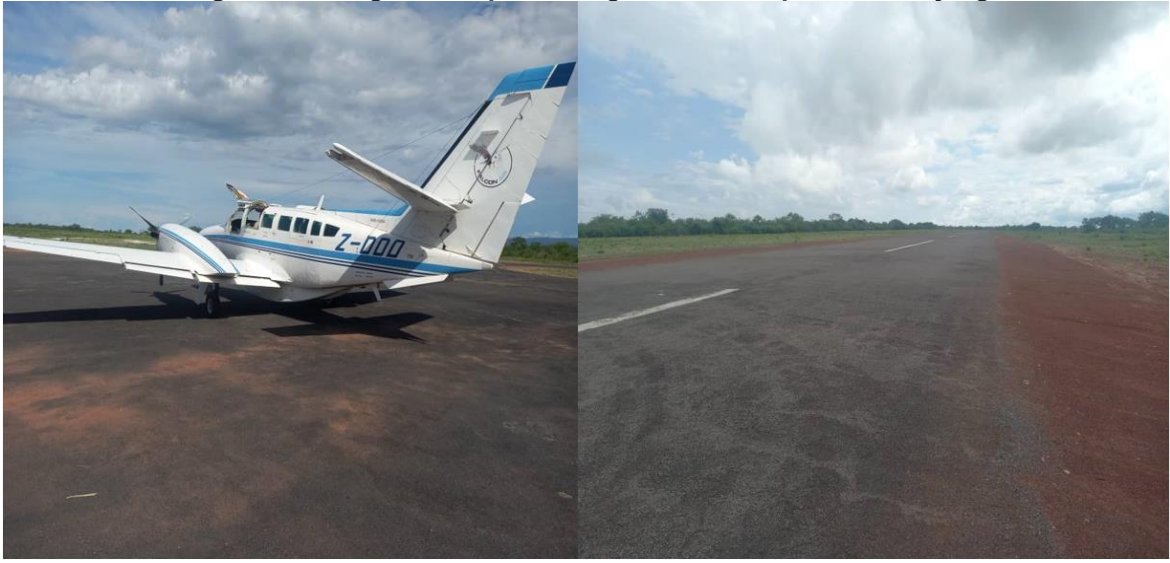
Figure 27: Binga Airstrip awaiting concrete asphalt overlaying
