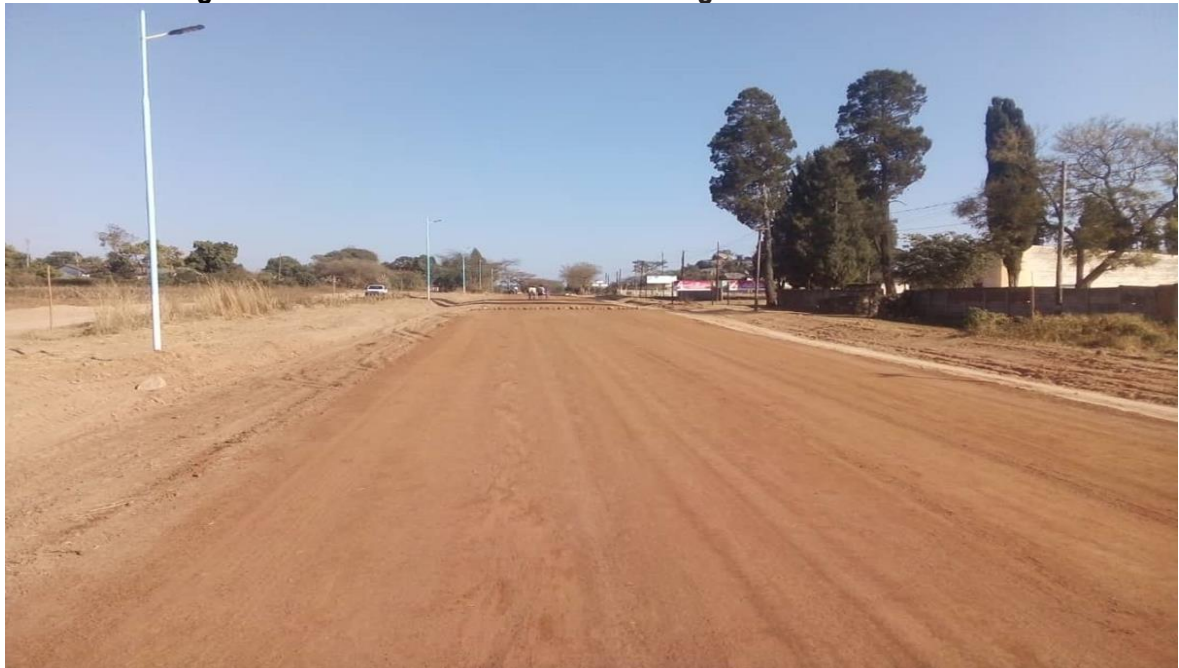
Figure 24: Monte Cassino Road Surfacing- Marondera District
