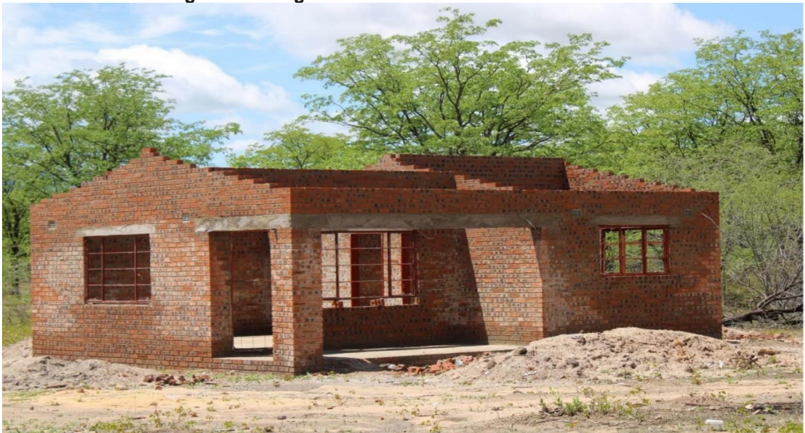
Figure 36: Binga Flood Victim house under construction.
