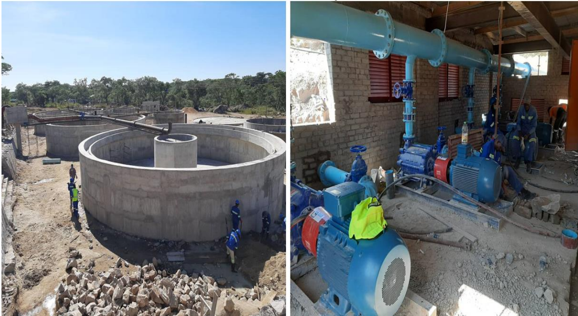
Figure 32: Construction of sedimentation tanks and mounting of pumps and motors at Chivhu water treatment plant
