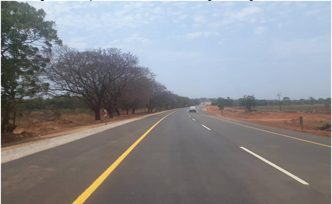
Figure 23: Completed section of Harare-Masvingo-Beitbridge Road
