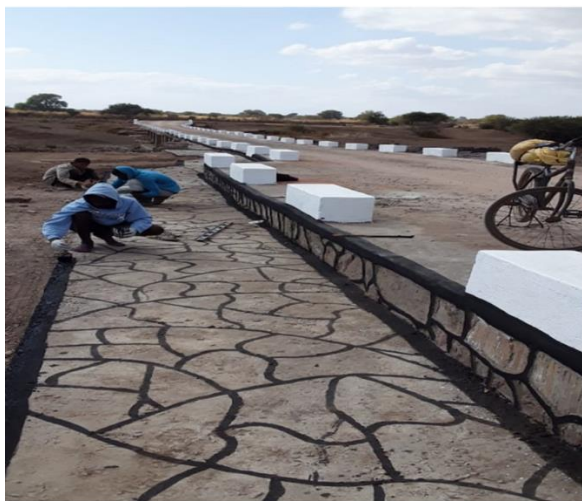
Figure 25: Maphani Bridge rehabilitation- Beitbridge District
