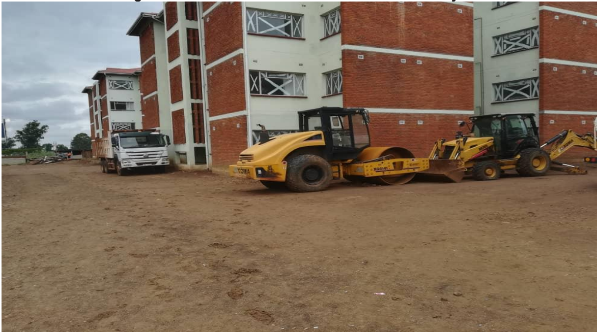
Figure 33: ZRP Chimoio Flats civil works underway
