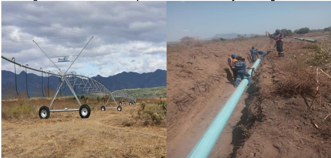
Figure 5: Centre Pivot and Pipeline Installation at Kanyemba Irrigation Scheme
