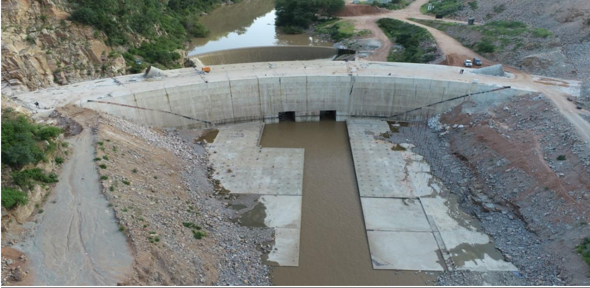
Figure 30: Construction of Gwayi-Shangani dam
