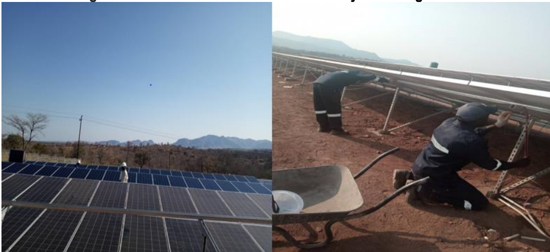
Figure 7: Solar Powered Installation at Kanyemba Irrigation Scheme
