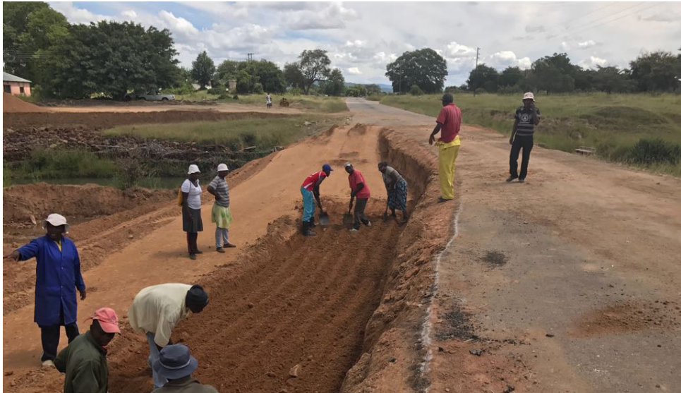
Source: Department of Roads
