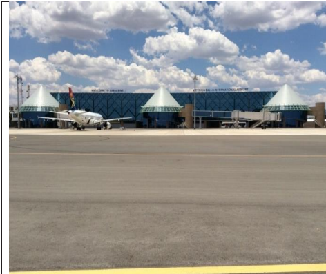
New International Terminal Building from the Airside
