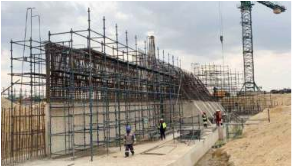
Mbudzi Interchange Bridge
