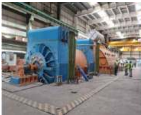
Installed steam turbine and generator for unit 7
