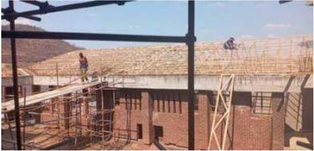
Gwanda Magistrates Court under construction
