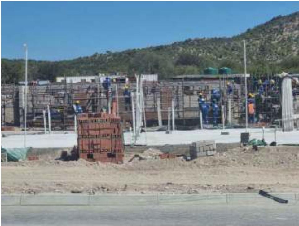
Staff Houses and road under construction at Beitbridge Border Post
