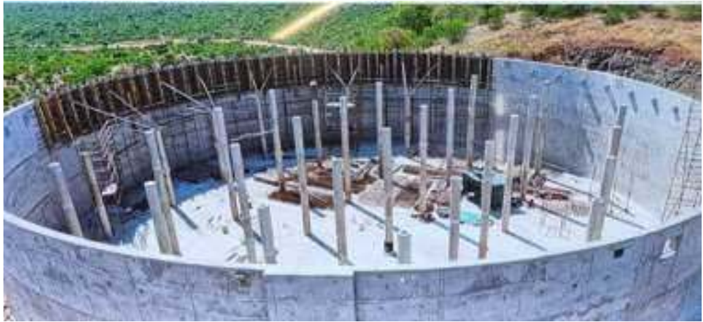
Megalitres reservoir superstructure is awaits roofing and other ancillary works
