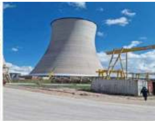
Cooling tower for units 7 & 8
