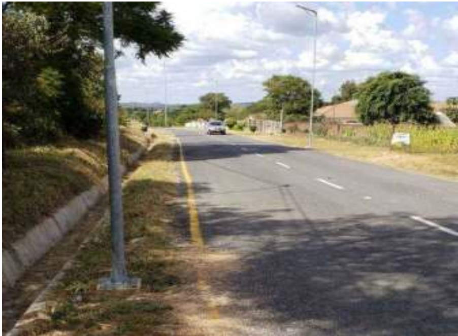
Camperdown Road resurfacing completed on 2km stretch
