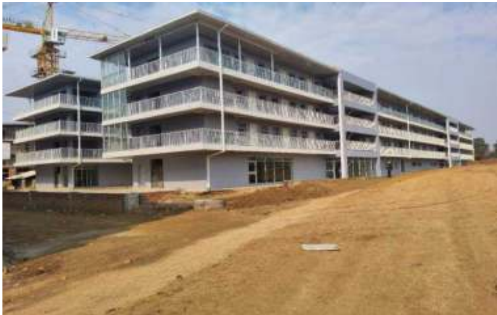
Bulawayo Student Accommodation Complex Completed Block
