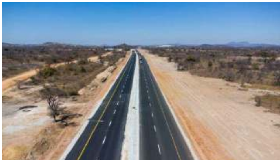
Part of the 20km Masvingo Urban along Harare-Masvingo-Beitbridge road
