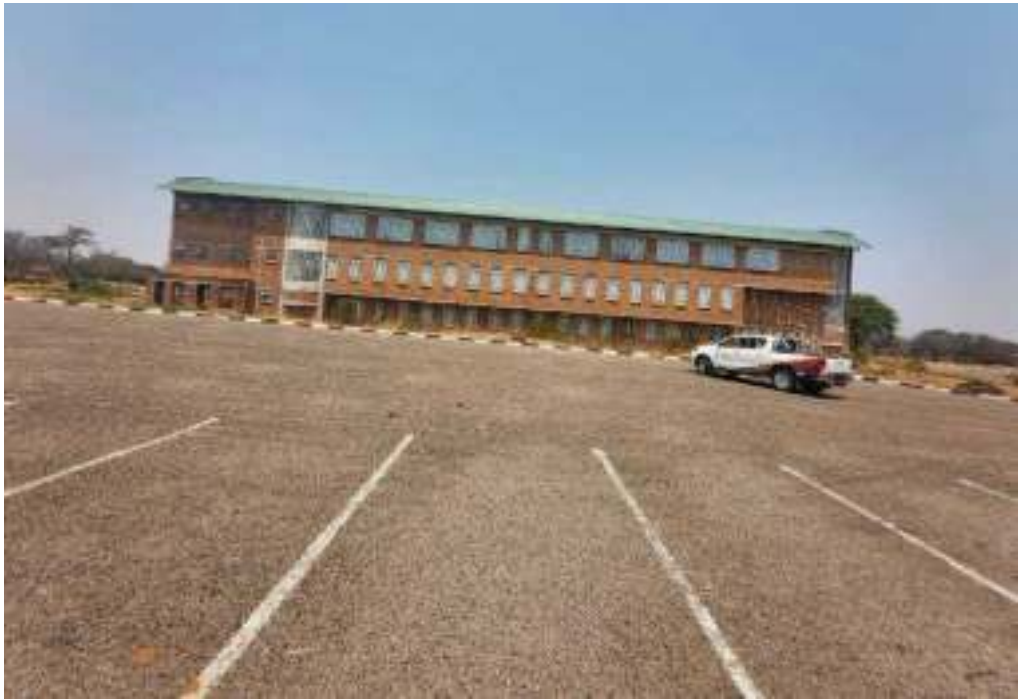
Lupane Provincial Composite Office Block
