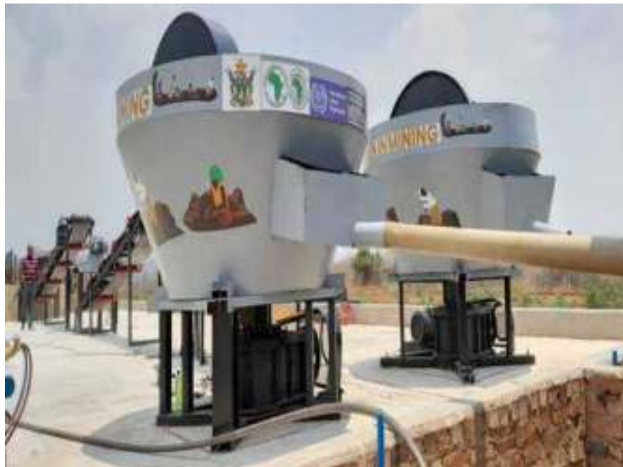
Guruve Gold Milling Plant, 95% complete.
