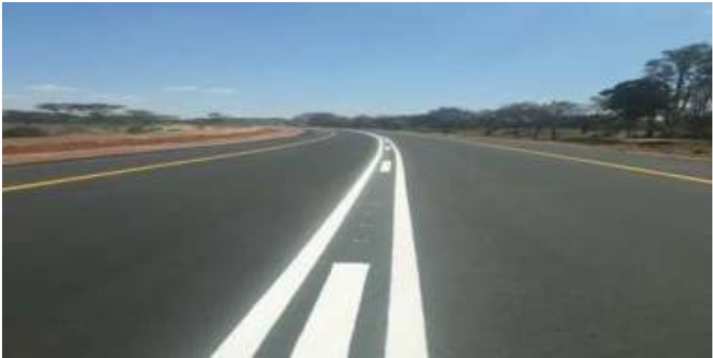
Section of the completed Beitbridge-Harare Road
