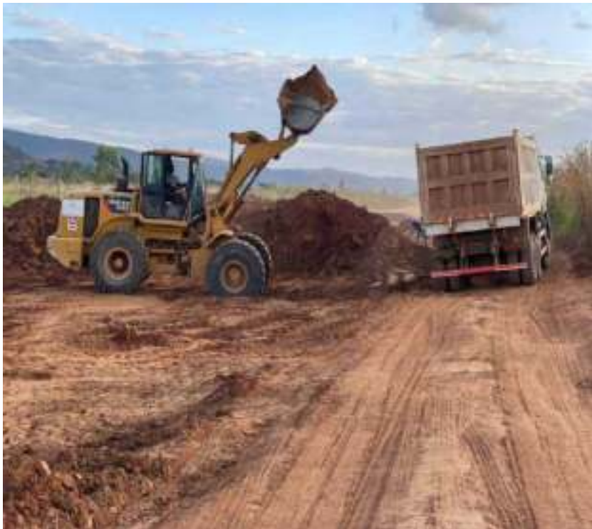
Matepatepa Mountain side road under construction
