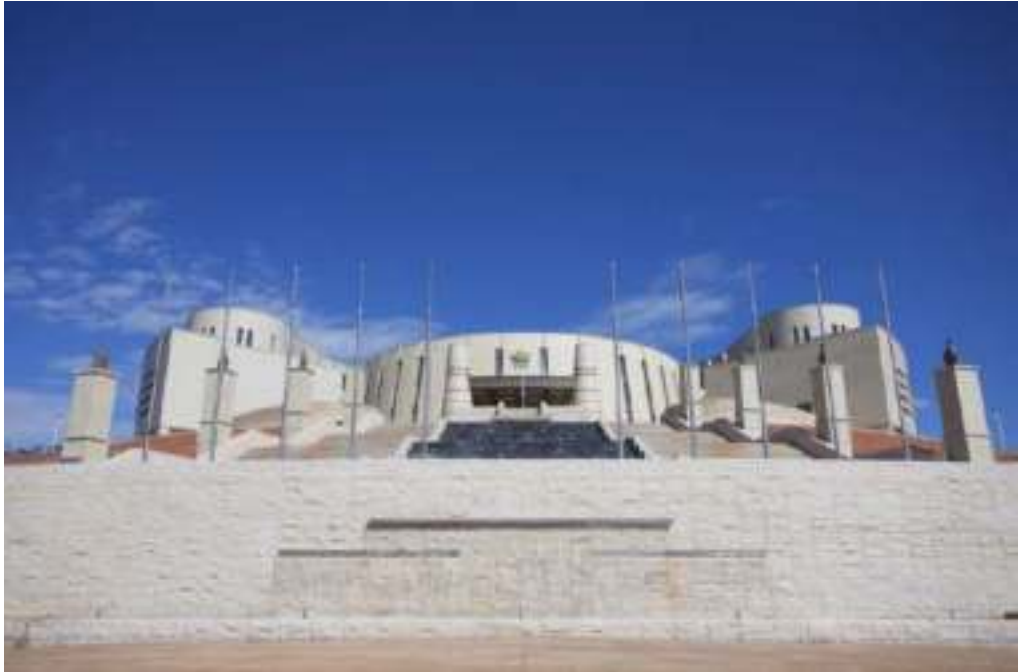
Completed New Parliament Building
