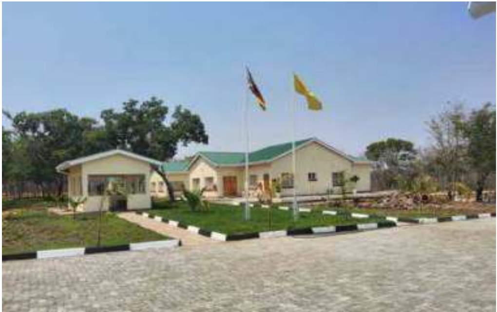
Recently completed Lupane Magistrates Court
