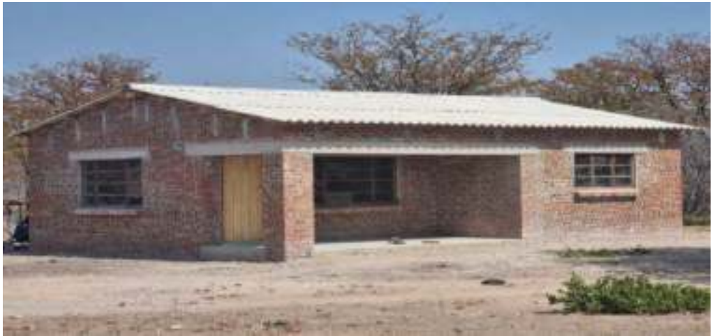
Completed Binga Flood Victim house
