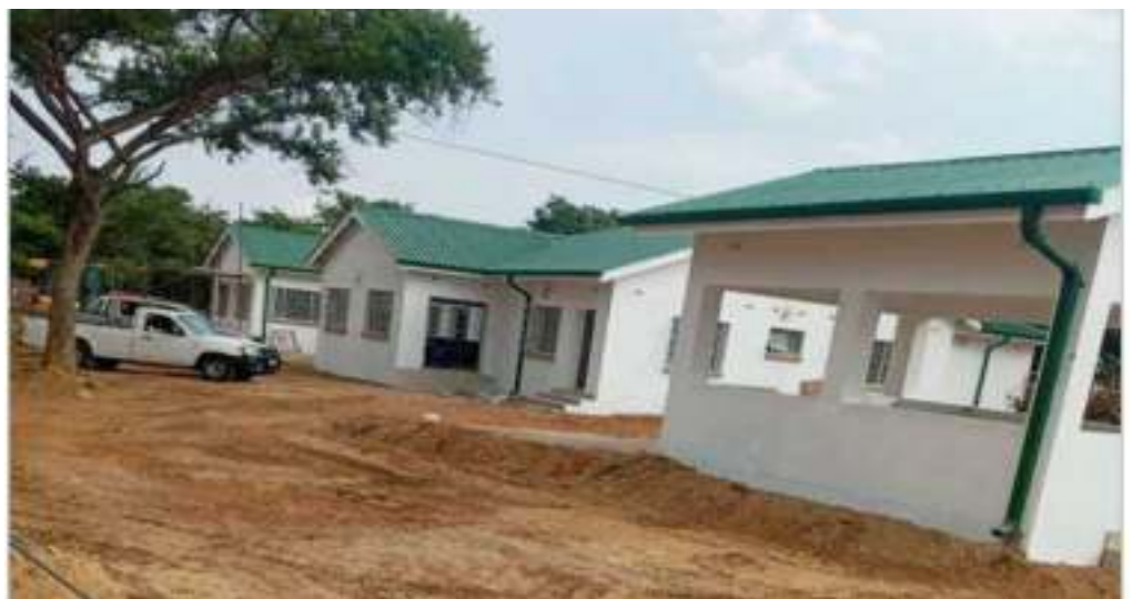
Completed Epworth Magistrate Court
