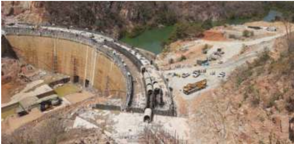
Construction of Gwayi Shangani Dam
