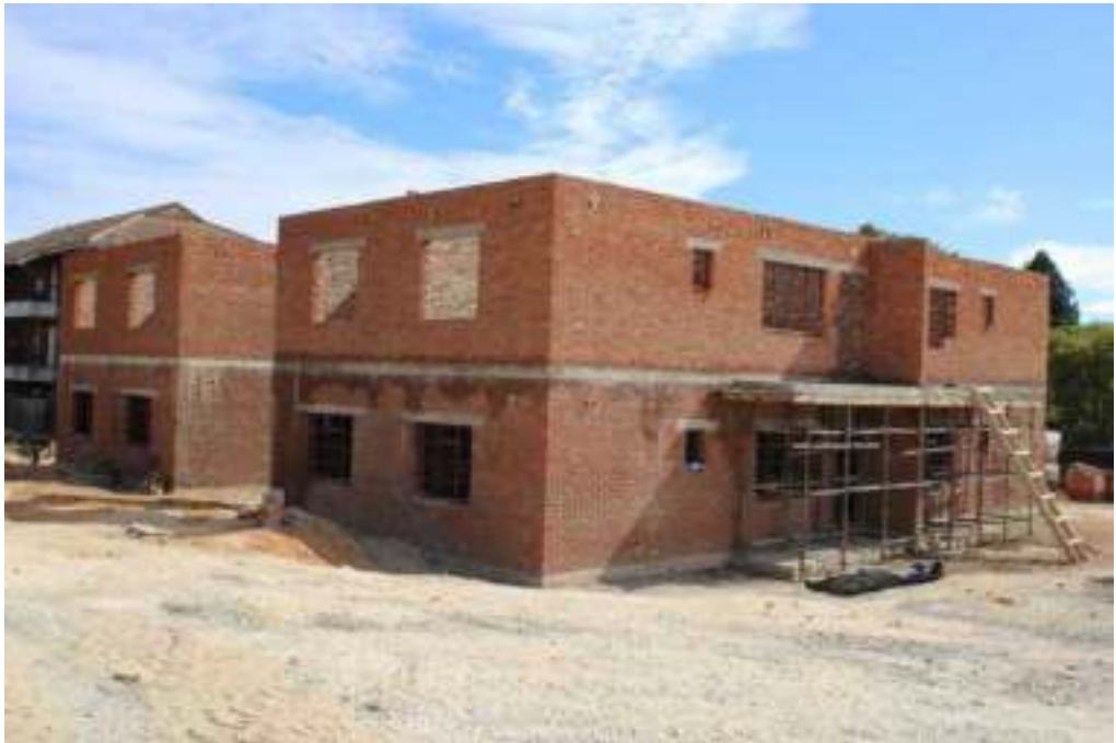
Block of flats under construction in Marondera
