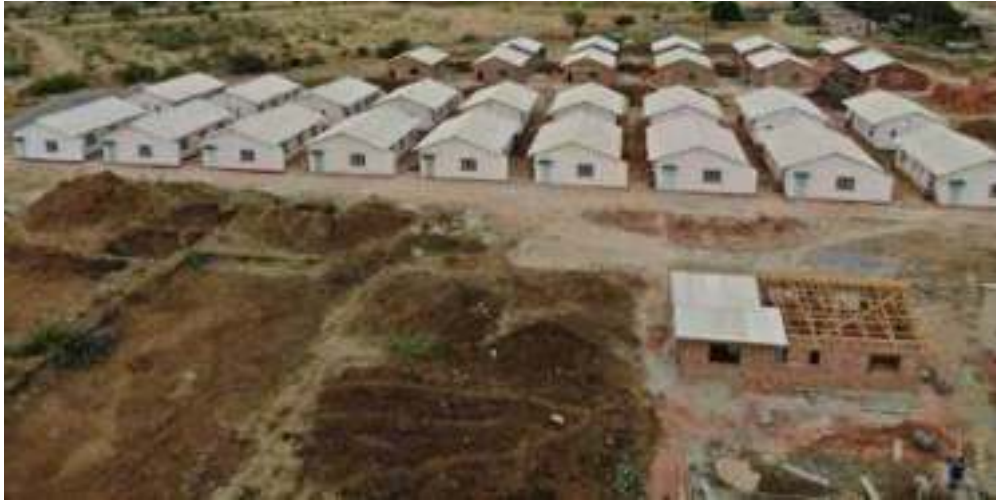
Housing Units at Dzivarasekwa under construction
