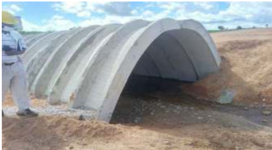
Bridge works at Harare-Mutare Road Dualisation Project – Melfort section
