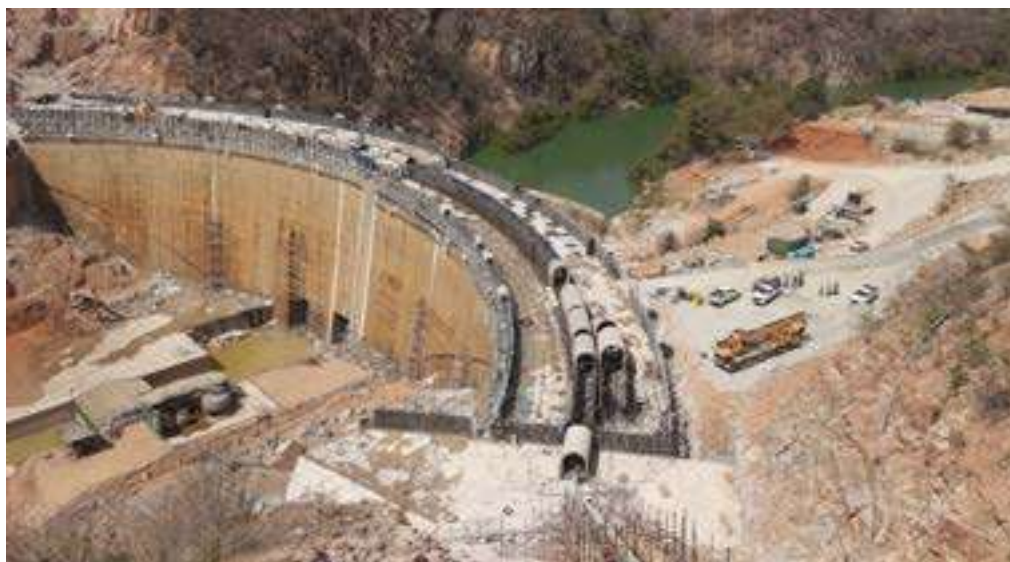
Gwayi Shangani Dam
