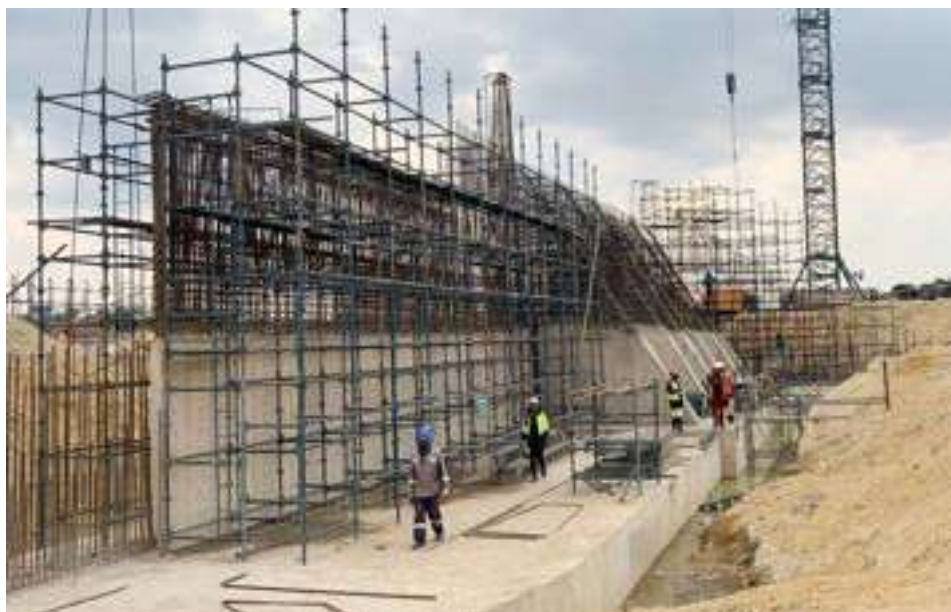
Mbudzi Interchange Construction
