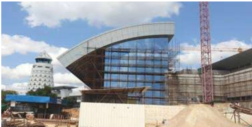
Outside of the Terminal Building
