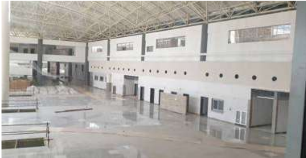
Inside of the Terminal Building
