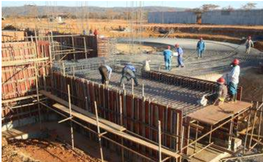
Construction at Manhize
